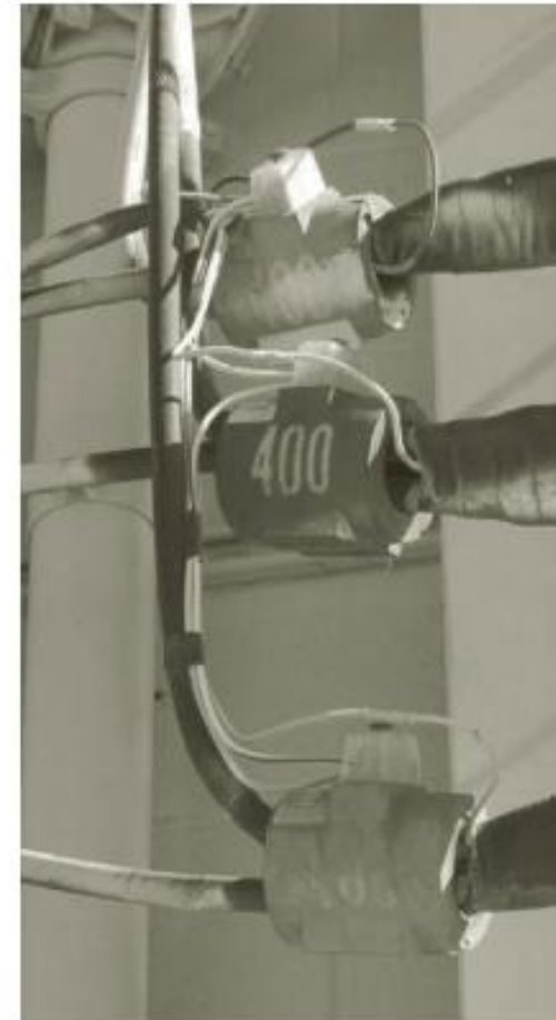
FIGURE 2-17 The incoming power line is inserted through the opening in the transformer.
