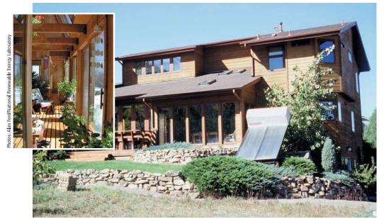
FIGURE 16.9 This passive solar home (right) in Golden, Colorado, collects and stores incoming solar energy to provide much of its heat in a climate with cold winters. Notice the solar hot water heating panels in the yard. Some passive solar houses have sunrooms (see inset photo) to help collect incoming solar energy.
