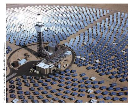
**FIGURE 16.12** Solar thermal power: In this system in California an array of mirrors tracks the sun and focuses reflected sunlight on a central receiver to boil the water for producing electricity.
